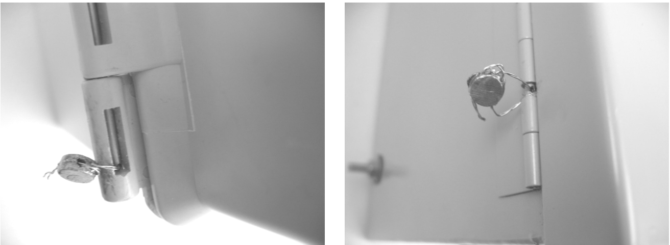
Figure 2.4—Seal wire installation on an 1141C hinge (left) and an 1141L hinge (right)
