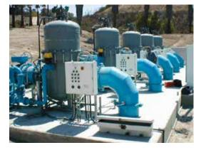
Model 2596 fabricated automatic self-cleaning pipeline strainers are available from 10" to 60" I/O sizes with continuous flow,
