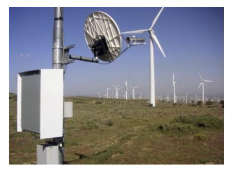
Highly reliable advanced satellite telemetry is used in the remote regions that some wind turbines inhabit.
