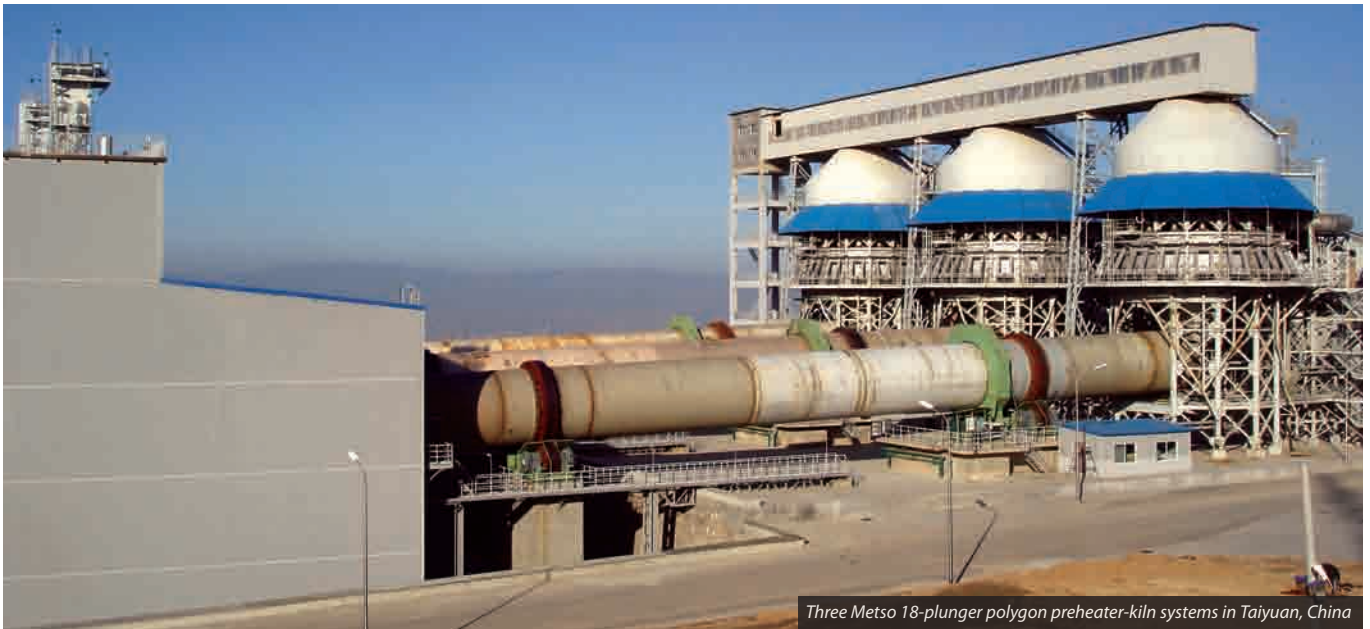
Three Metso 18-plunger polygon preheater-kiln systems in Taiyuan, China
